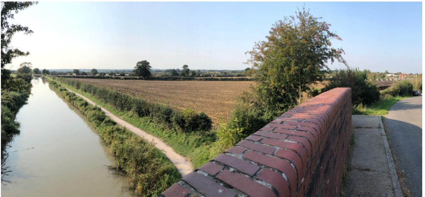
Photograph from canal bridge facing westwards - September 2020
